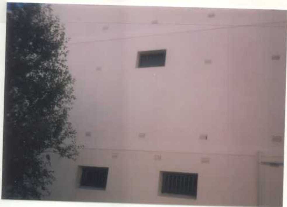
Breakwater - prev. prison, now hotel
